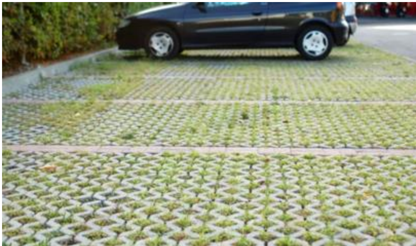
Figure 5: An example of permeable parking spaces.
